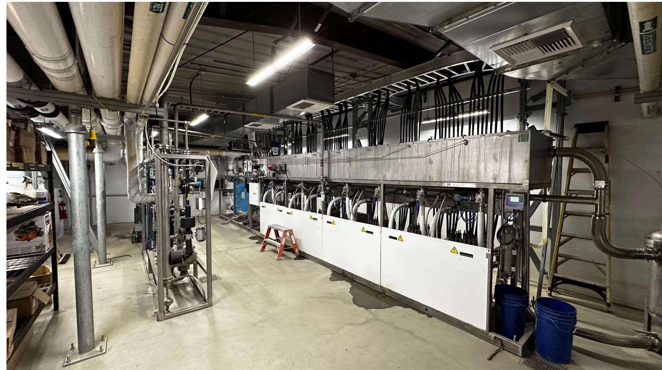
Image of Nel's Proton Exchange Membrane (PEM) Electrolyzer System including 8 fuel cell stacks.
